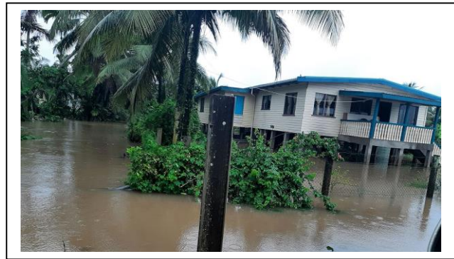
Figure 27: Flooding at Vuci Irrigation road on October 8, 2019. Photo: Supplied to Fiji Times.
